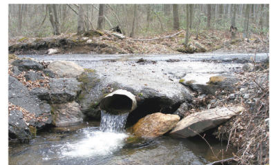
Discharging sewage in canals
